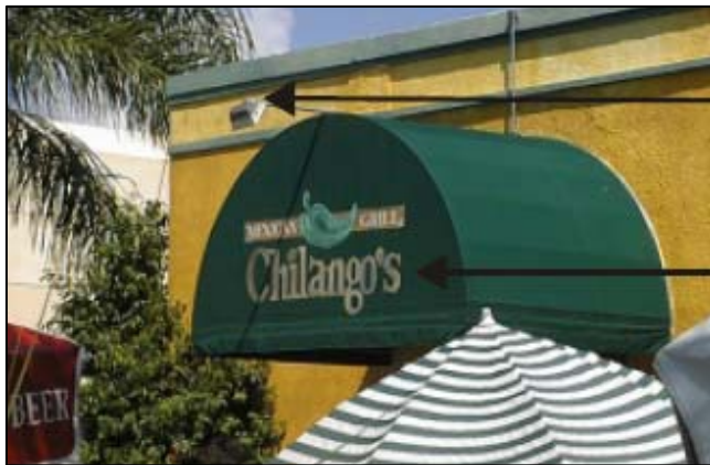
Sign painted on the face of a canvas awning over entry and lit discreetly by external lighting.
