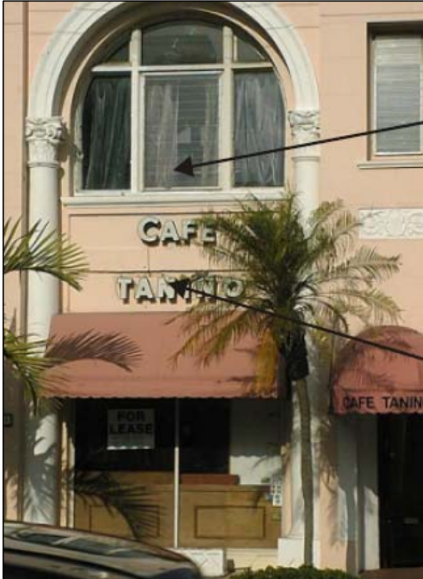
The sign is centered within the symmetrical arrangement of the window above and shopfront below and has internally lit letters.
