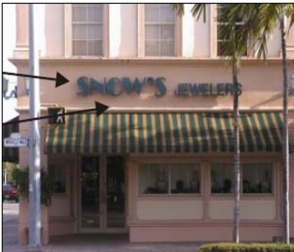
The sign runs horizontally along the expression line and has internally lit letters.
