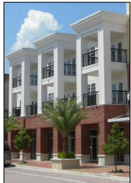
Tuskawilla Road Colonnade Winter Springs Town Center
