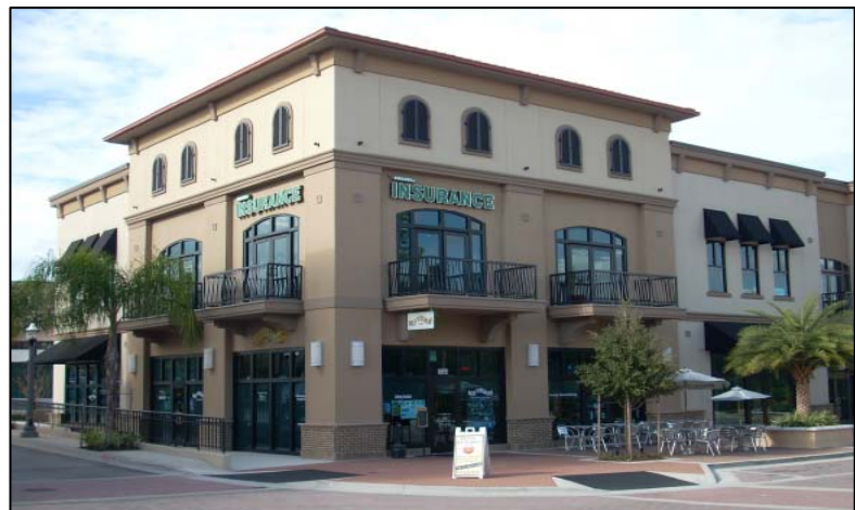
Tuskawilla Road Balconies; Winter Springs Town Center
