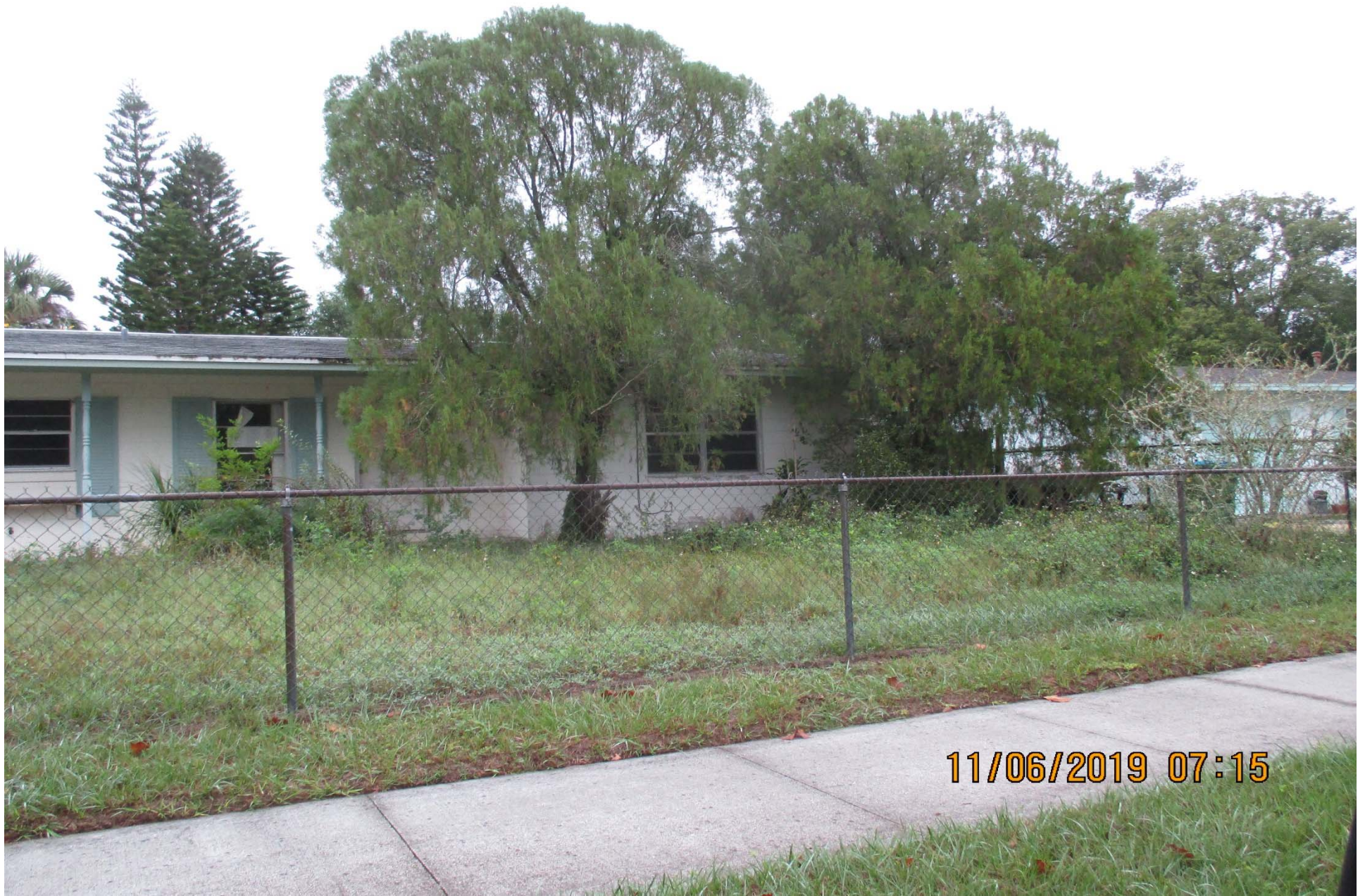
Grass Overgrown on 11/06/19
