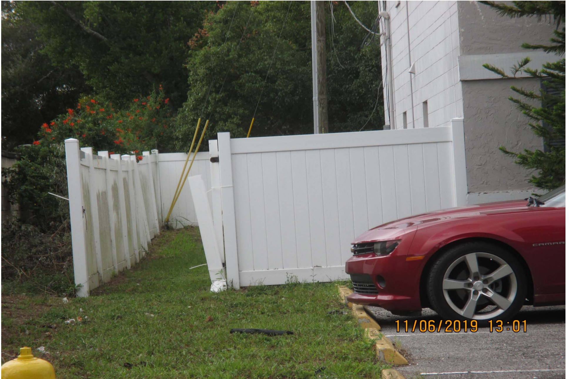
Fence broken and green growth on the all over Trash in the front yard 11/06/19
