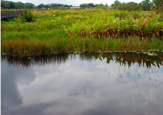
Figure 8. Oviedo Drainage and Stormwater Management & Erosion Control
