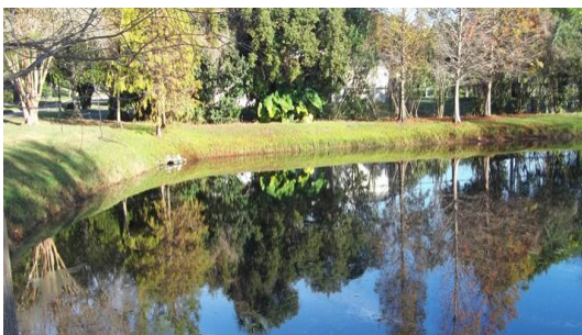
Stormwater pond located in Altamonte Springs.
