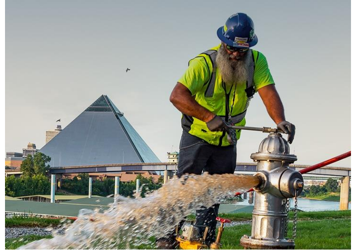
Figure 4. Hydrant Flushing in Memphis TN
