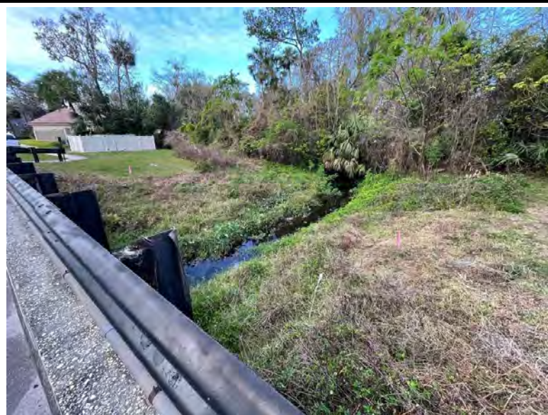
West of Sheoah Boulevard roadway crossing (facing south), remove sediment deposit
